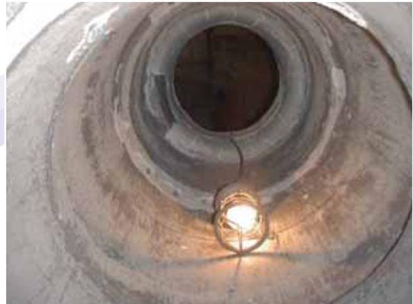
Figure 26b Casting filtered
