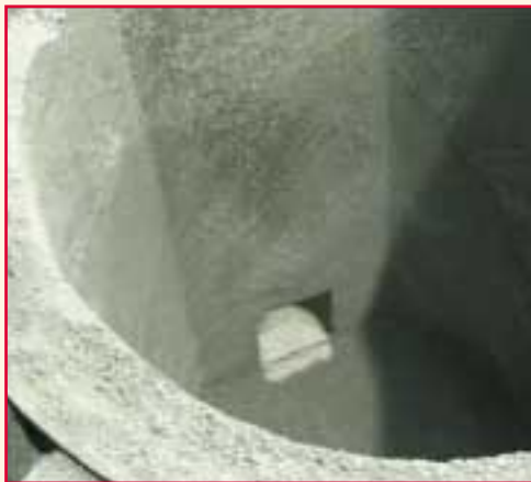
Figure 5: The finished KALTEK ISO lining
