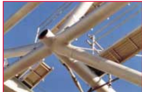
Figure 3: Casting cluster with cross-struts
