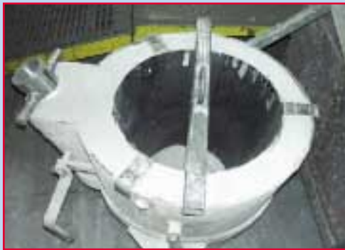
Figure 4: The void between the ladle and the shell has been filled with KALTEK ISO
